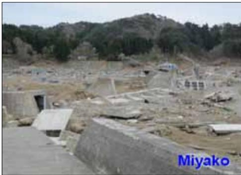
**Figure 1:** The 10m seawall was destroyed in Taro district, Miyako City, Iwate Prefecture [1]
