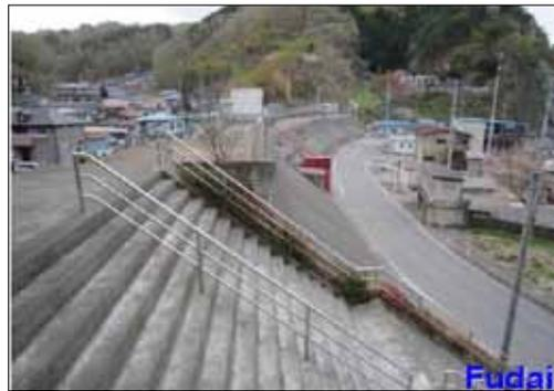
**Figure 2:** The 15.5m-high seawall was left intact in Ootabe district, Fudai village, Iwate Prefecture [1]
