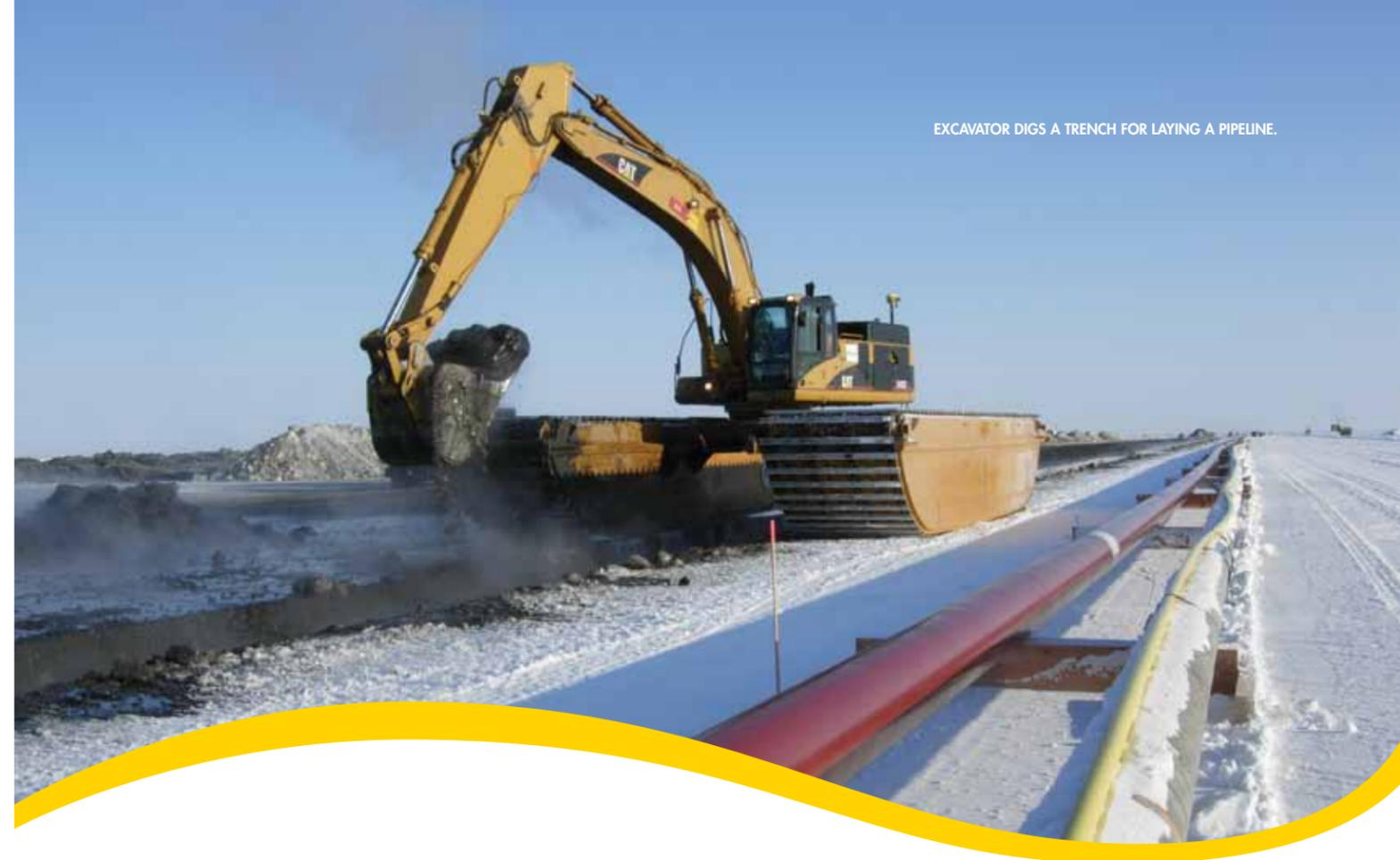
EXCAVATOR DIGS A TRENCH FOR LAYING A PIPELINE.
