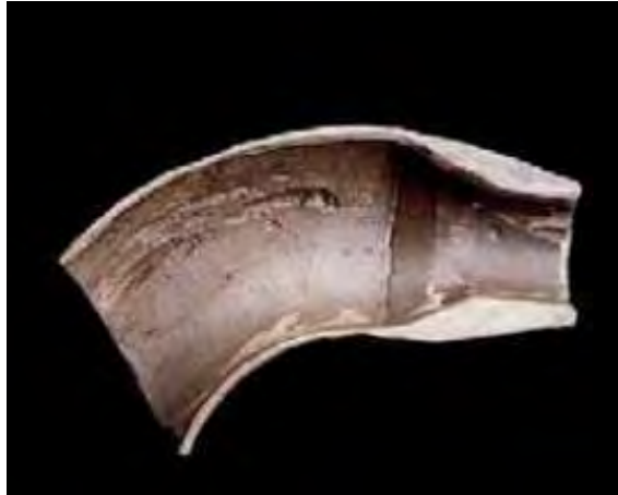
Figure 8: Erosion of a Pipe Bend
