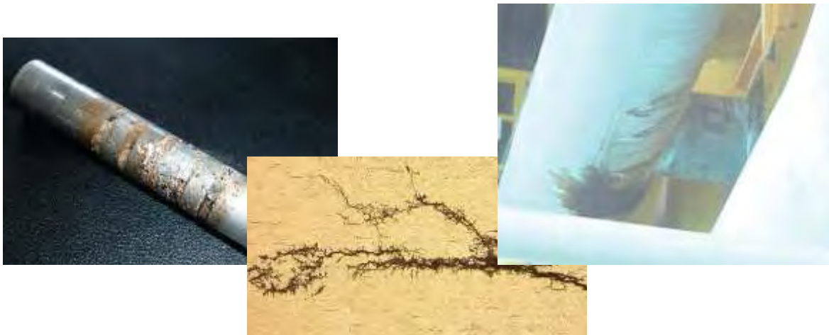
Figure 7: Examples of Stress Corrosion Cracking
